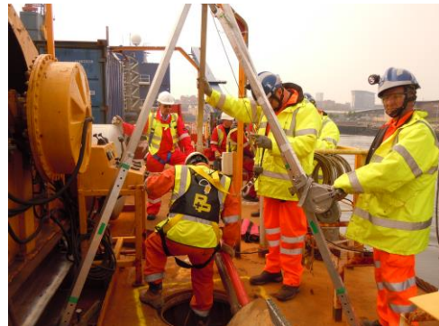
Man access into a 'Barge Tank'
