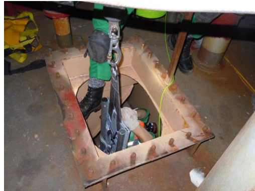
Entrance to a 'Coffer Dam'
