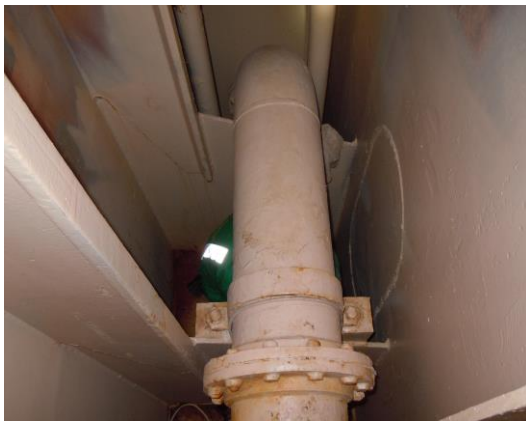
Plate 6: Casualty located under 300mm pipe
