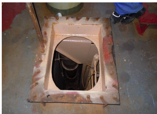
Plate 4: Access to No 4 Tank from deck level
